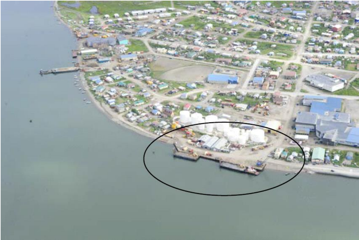
Kotzebue barge landing bulkhead
