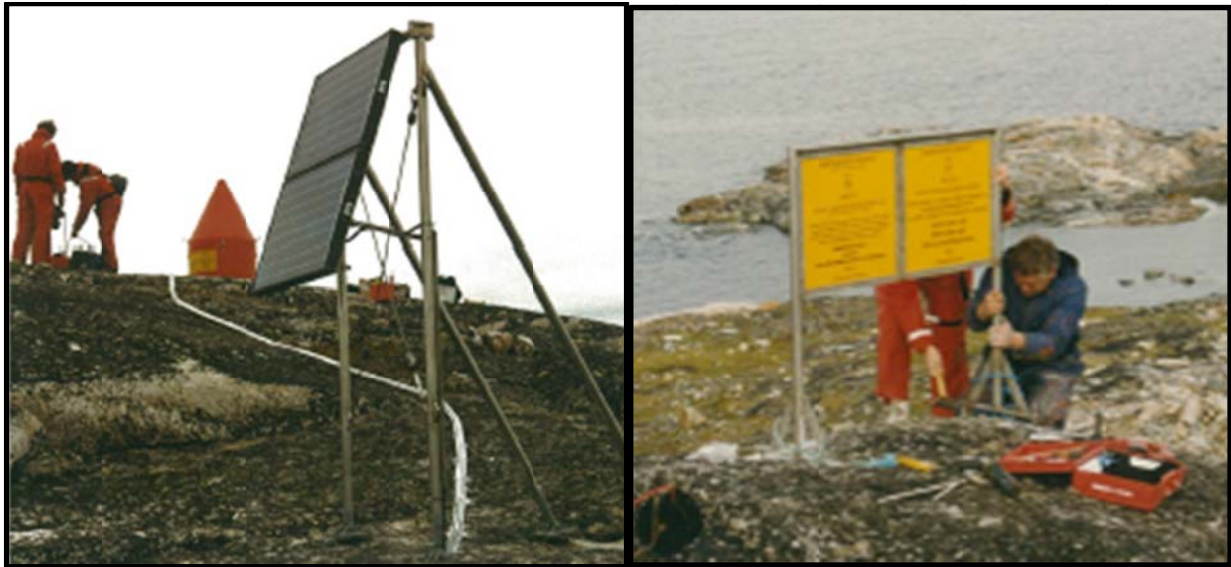
Figure 7 Example of cable protection against wild animals & notices to deter vandalism
